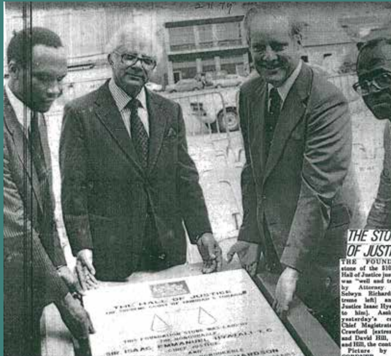
Laying of the foundation stone for the Hall of Justice. L-R: Attorney General Selwyn Richardson, Chief Justice Sir Isaac Hyatali, contractor David Hill and Chief Magistrate Roland Crawford (Trinidad Express, 1979)
