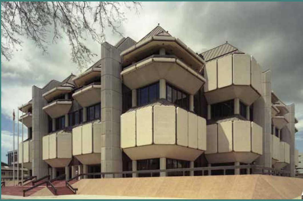
The actual building of the Hall of Justice.
