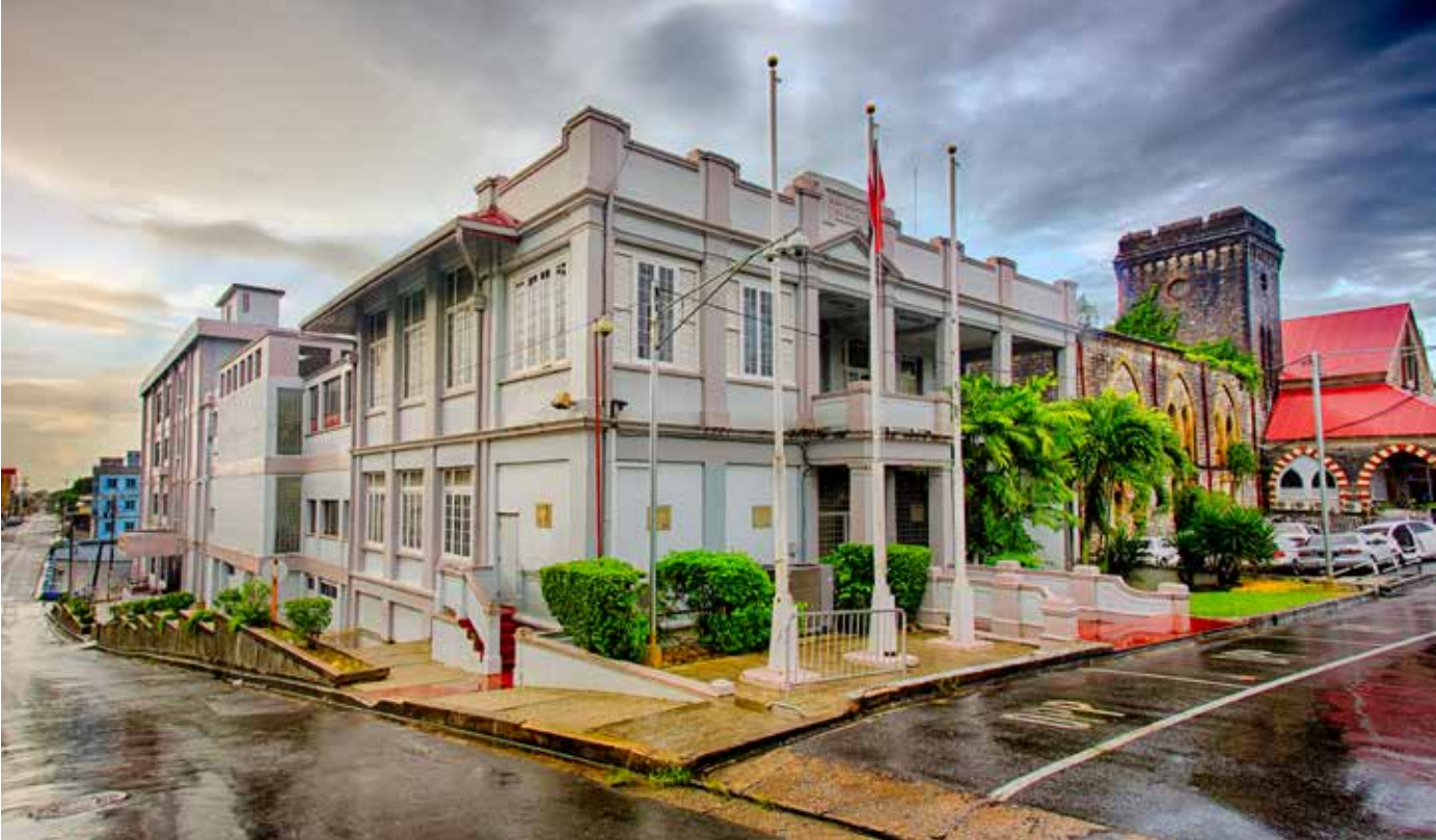
Supreme Court Buildings in San Fernando.
